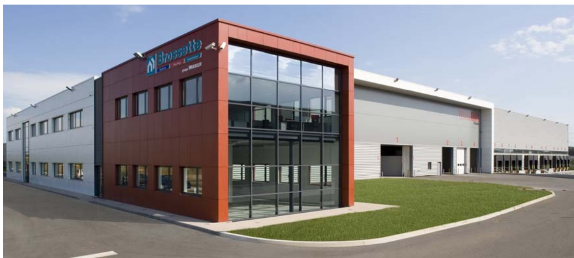
Montea 'More than warehouses' Brossette – Saint-Priest (Lyon) site
